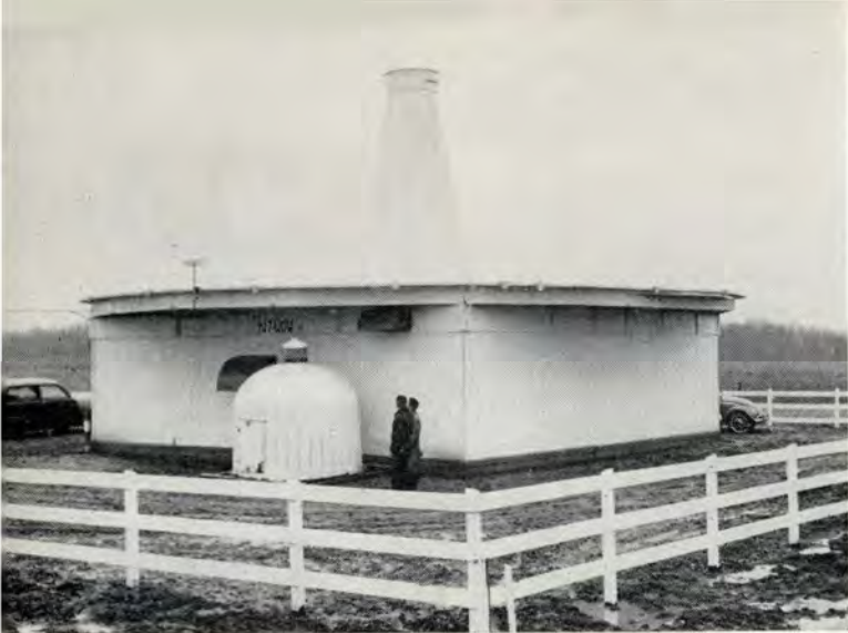
VORTAC installation, Herndon, Va., one of first of its type established by FAA. With proper receiving equipment, pilot gets precise direction and distance from transmitter. 260 units operate now. FAA plans 1100 installations by '65.
